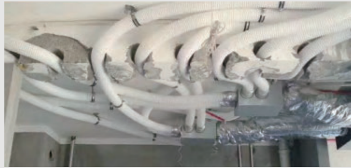
01-The holes in the house beams are quite large. ❌
